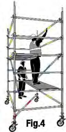
10. Relocate and stagger the temporary platform to nominally 1m above the ground. This platform will act as fall prevention. Install an access ladder through the opening section of platform – See Fig. 4.
